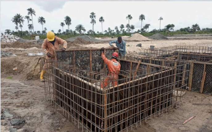
6 Celler Rig Matt and Fundation Job at UTA. A replacement OML Akwa Ibom State
