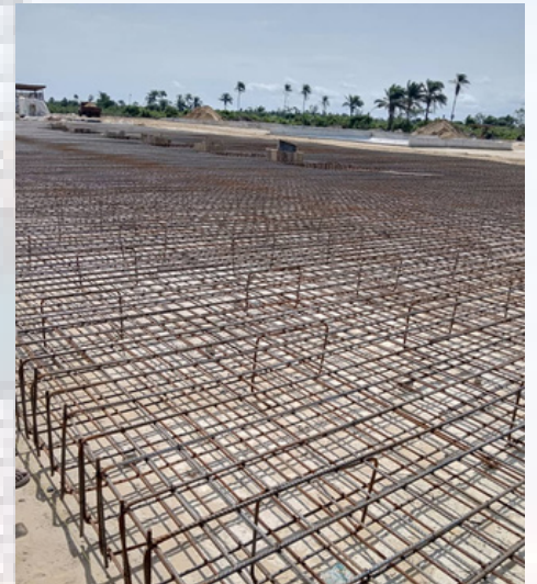
CSU Column Foundation job at EPF OML 13 Sterling Global Akwa Ibom State
