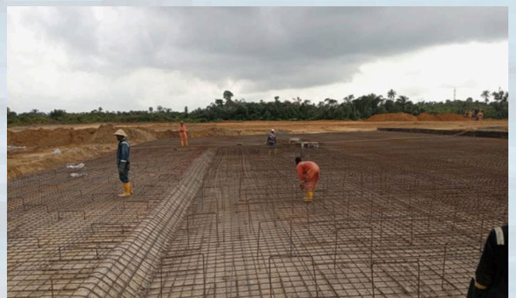
6 Celler Rig Matt and Fundation Job at UTA. A replacement OML Akwa Ibom State
