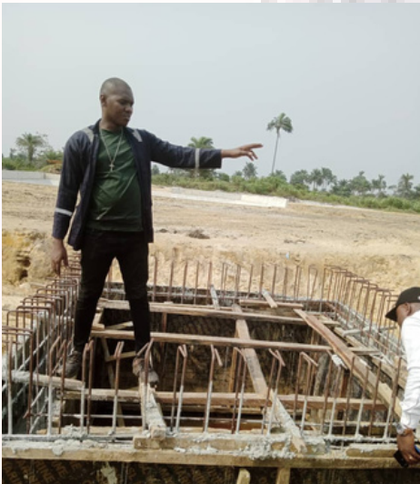
CSU Column Foundation job at EPF OML 13 Sterling Global Akwa Ibom State
